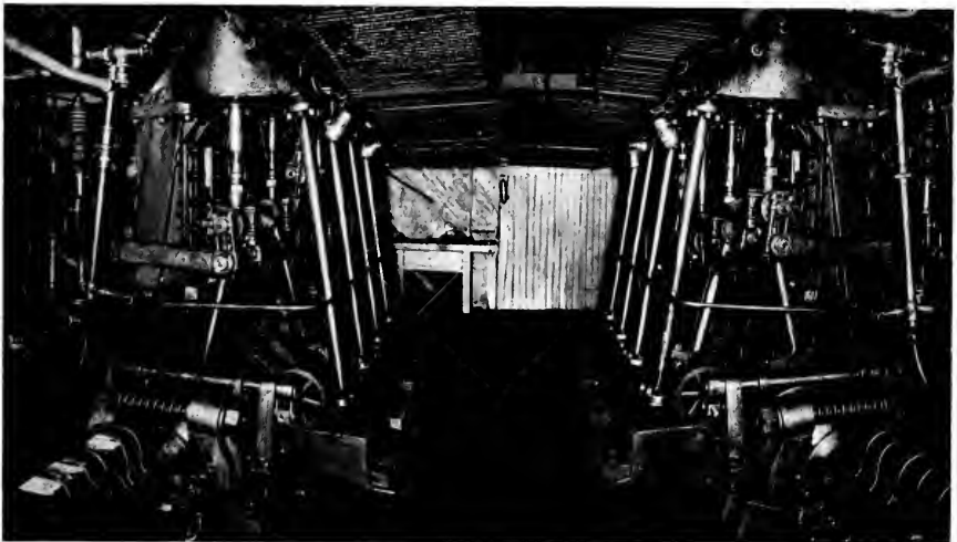
The engine-room of the motorship "Santino," stripped of ladders to show her Sumner Diesel engines. These engines rendered a splendid account of themselves on the long voyage from Puget Sound to Boston, and the makers of this Seattle product are highly gratified at the success attained.
